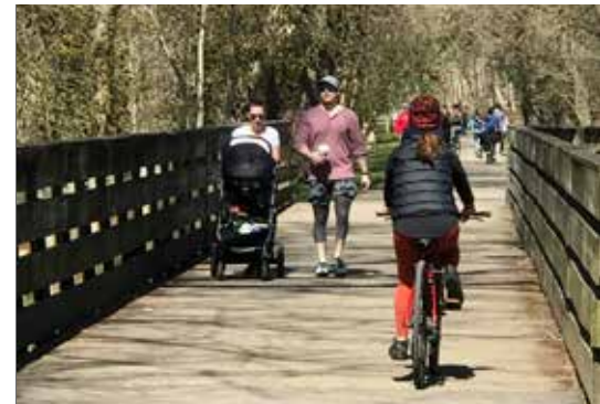
NISBET PARK BRIDGE
